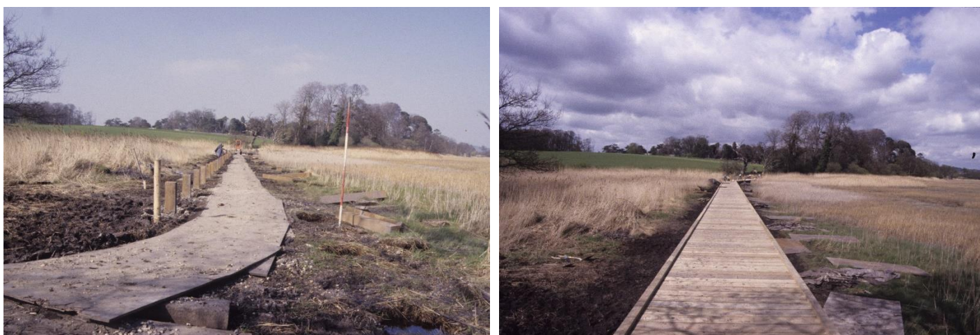
Fig. 8 – Boardwalk under construction and on completion c 1987/8 showing degree of trampling and ground disturbance
