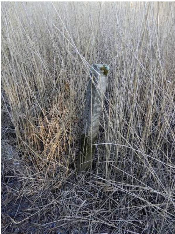
Fig 10 Concrete fence post in reed bed
